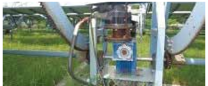
Figure 5: Tracking system of PTC
