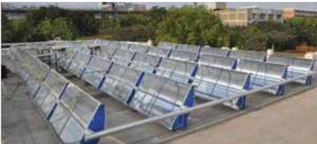
Figure 3: PTCs with different sizes and types of reflectors
