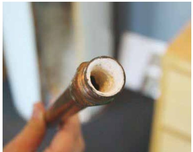
Figure 7: Scaling of inner lining of pipe
