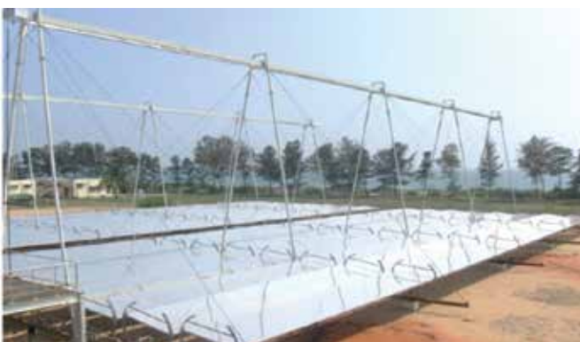
Figure 1: Linear Fresnel reflectors
